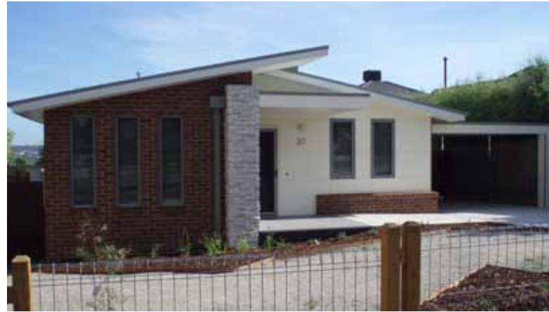
Pre-fabricated housing 8 weeks from start to finish.
