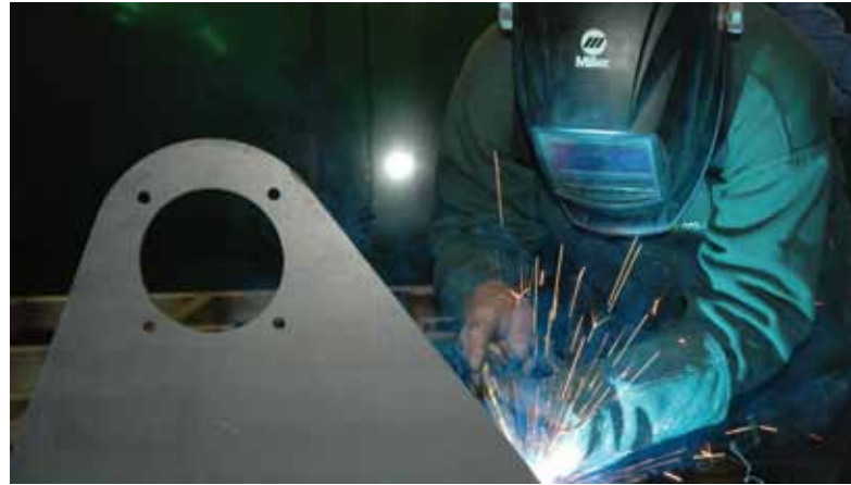
Welding the Airchange air conditioning and ventilation units
